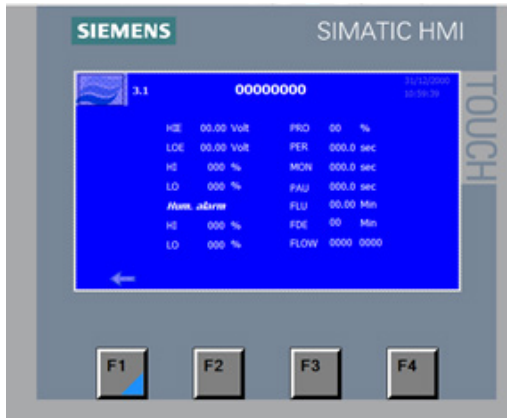
Display 3.1 - Zone controller
